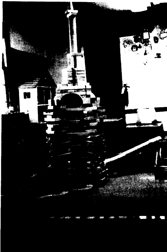
FIGURE I.2. Photograph of Block Construction
